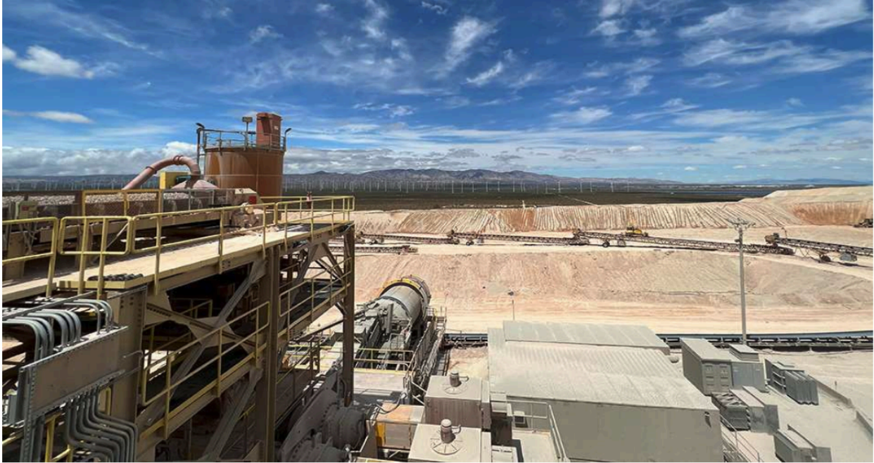
Soledad heap Leach operations
